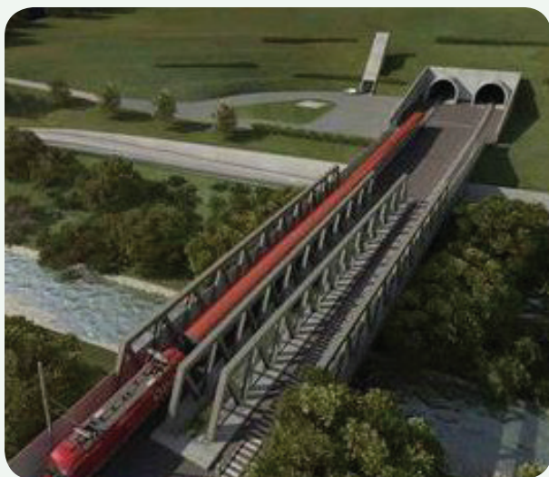
Access to the Semmering Base Tunnel
