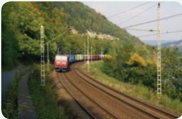
View of existing track in the Elbe Valley works
