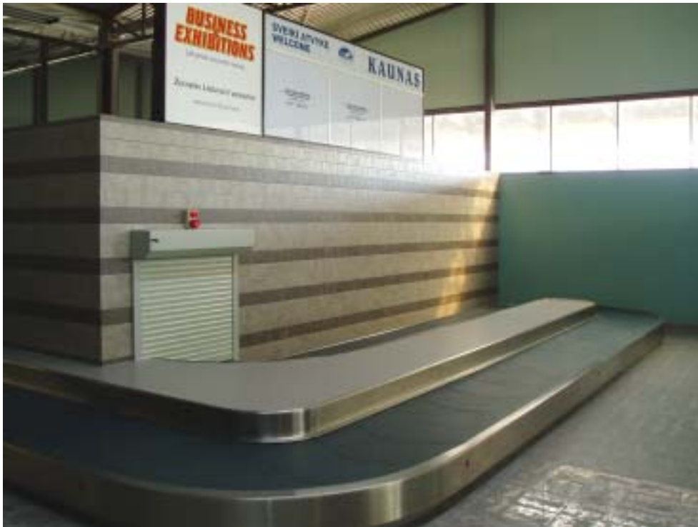
The baggage reclaim unit. Note the security shutters, which house an inbound X-Ray machine for the hold baggage.
