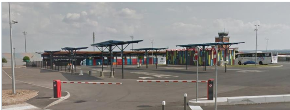
Figure F.36: the new bus and coach terminal at Beauvais-Tillé airport
