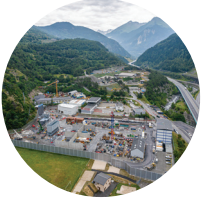
Lyon Torino Base Tunnel © Caroline Moureaux (Tunnel Euralpin Lyon Turin TELT)
