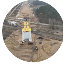
Rail Baltica mainline © LTG Infra I Rail Baltica
