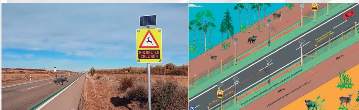
Illustration 52: Example of a warning system and channelling of animals on the road. Source: Regional Government of Castilla y León
