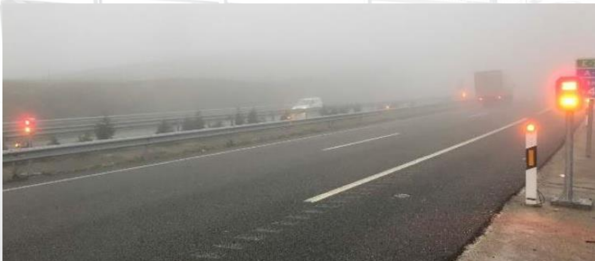
Illustration 39. Anti-fog system on the A-8 motorway. Source: DGT
