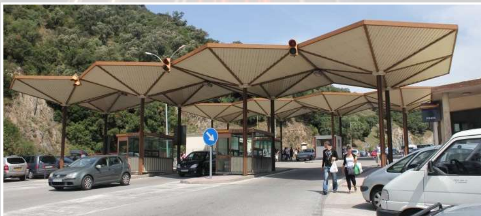
Figure 6 Le Perthus. Spain - France Border Crossing
