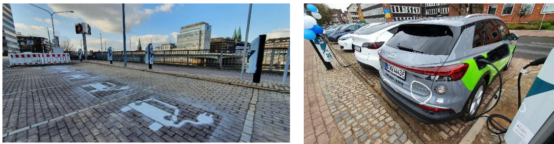
Charging hub in Bremen with six charging points at one grid connection (under construction and in use) (photos: Glotz-Richter)
