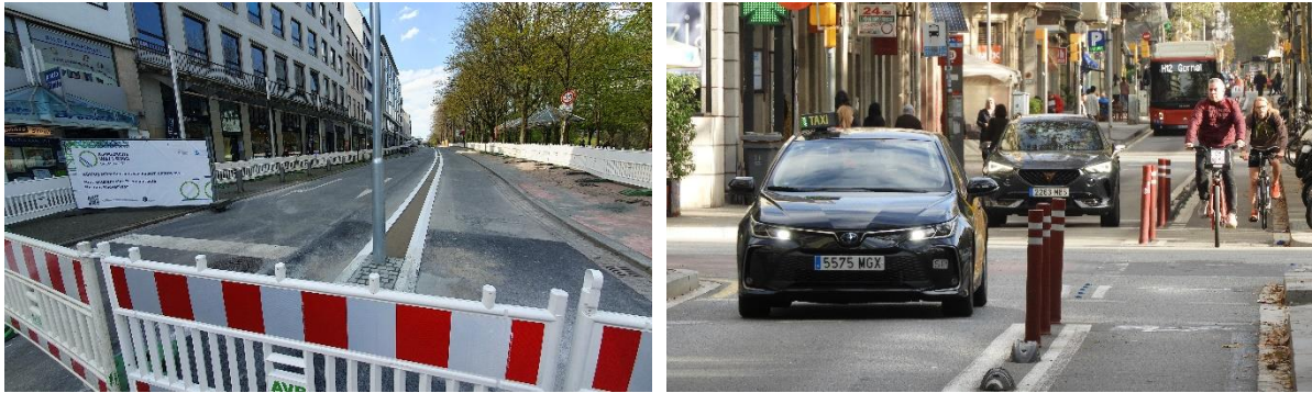
Graphs: Converting car lane into a bike lane (in progress Bremen; done Barcelona); photos: Glotz-Richter
