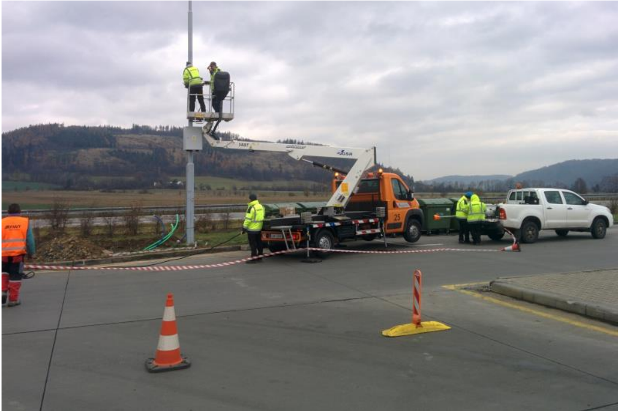
Figure 8 Installation of dynamic information equipment at Rest Area – pilot project
