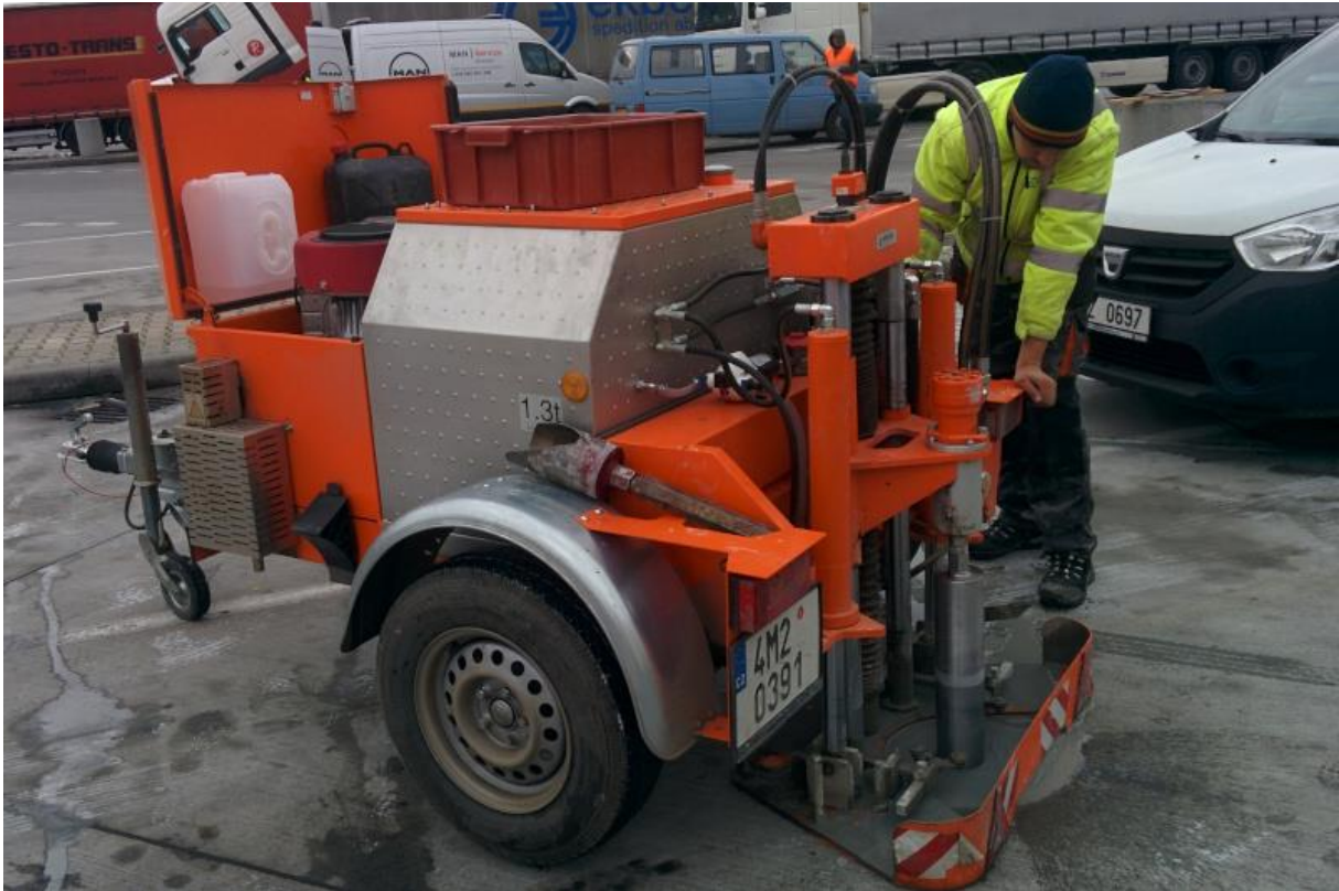
Figure 9 Installation of dynamic information equipment at Rest Area – pilot project
