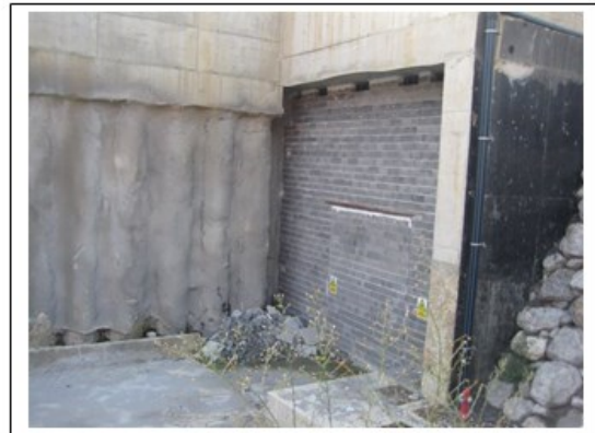
Ortuella side. The tunnel's exit is complete, although it has been temporarily closed for safety reasons.
