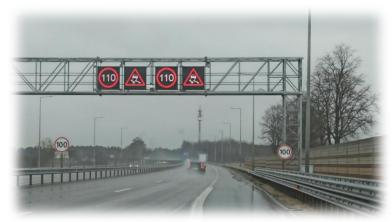
The SMWS consists of electronic variable message signs (VMS), weather condition sensors that monitor road surface conditions, temperature, wind speed, and other parameters, as well as traffic flow analysis devices that calculate traffic conditions at specific locations on the road.
