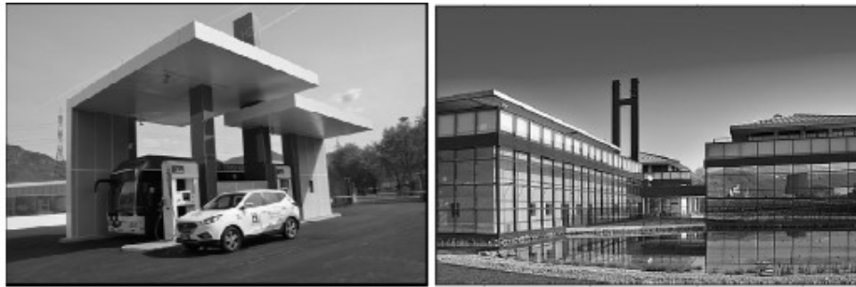
Figure 7: Bolzano hydrogen station
