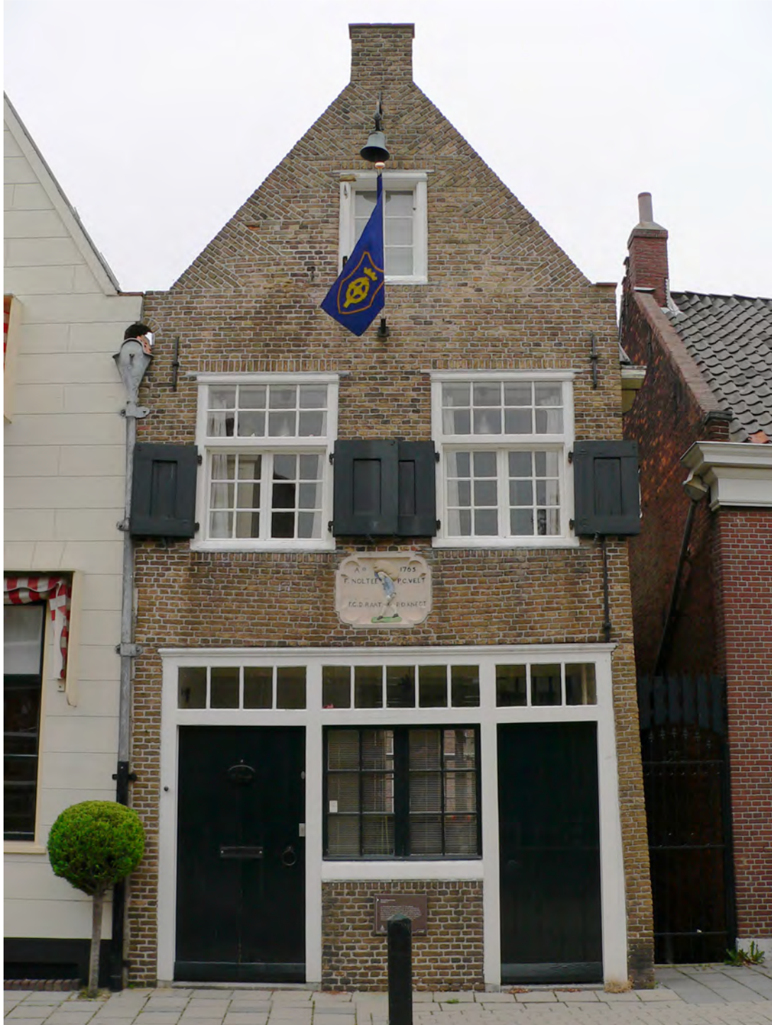
Figure 106. The porters' guild house at Maassluis from 1765 (photo by the author).
