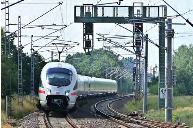
Picture: High speed train on the Berlin – Hamburg line near Paulinenaue (Source: www.wikipedia.de )
