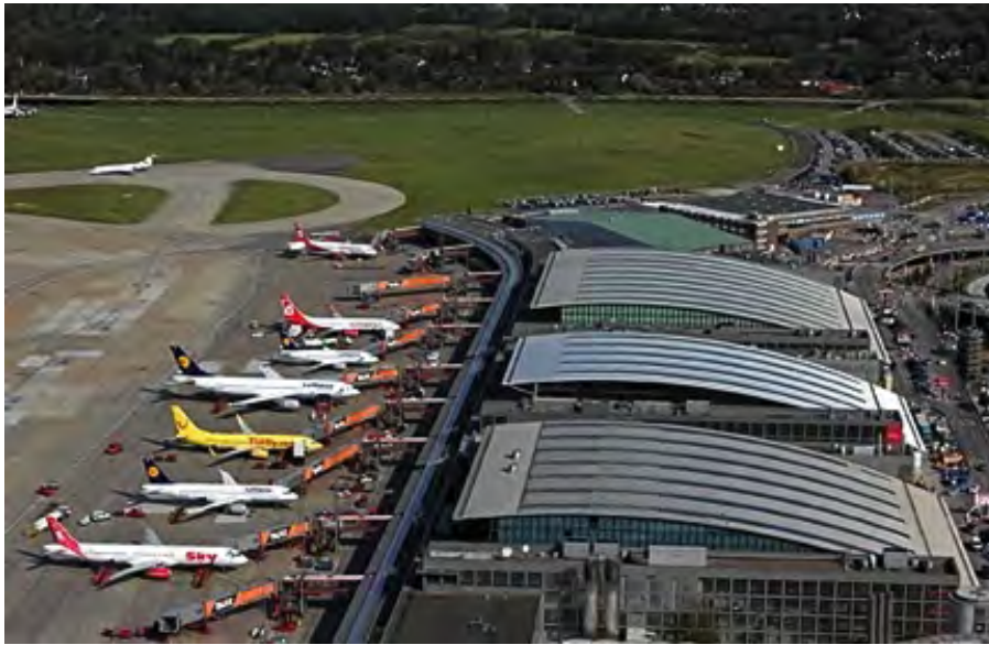
Picture: Hamburg International Airport – Overview (Source: www.wiki-pedia.de )
