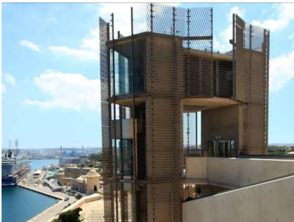
Below: The high capacity lift installed adjacent to the fortifications to link the Grand Harbour with Upper Valletta.
