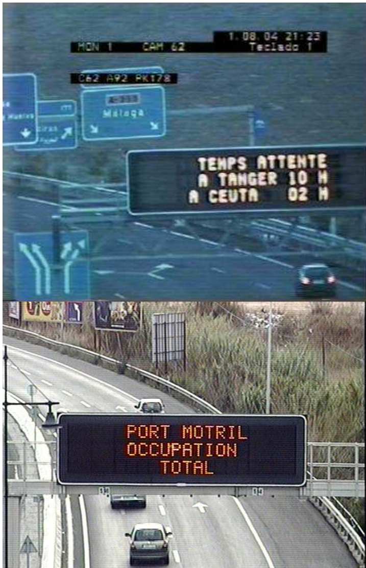
Figure 1: VMS displaying information on waiting times and parking places availability at sea ports.
