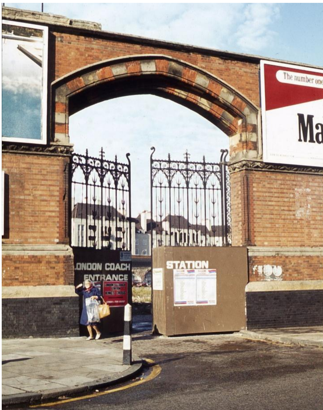
Figure 6.3: United Kingdom: improvised London coach station after 1985 deregulation
