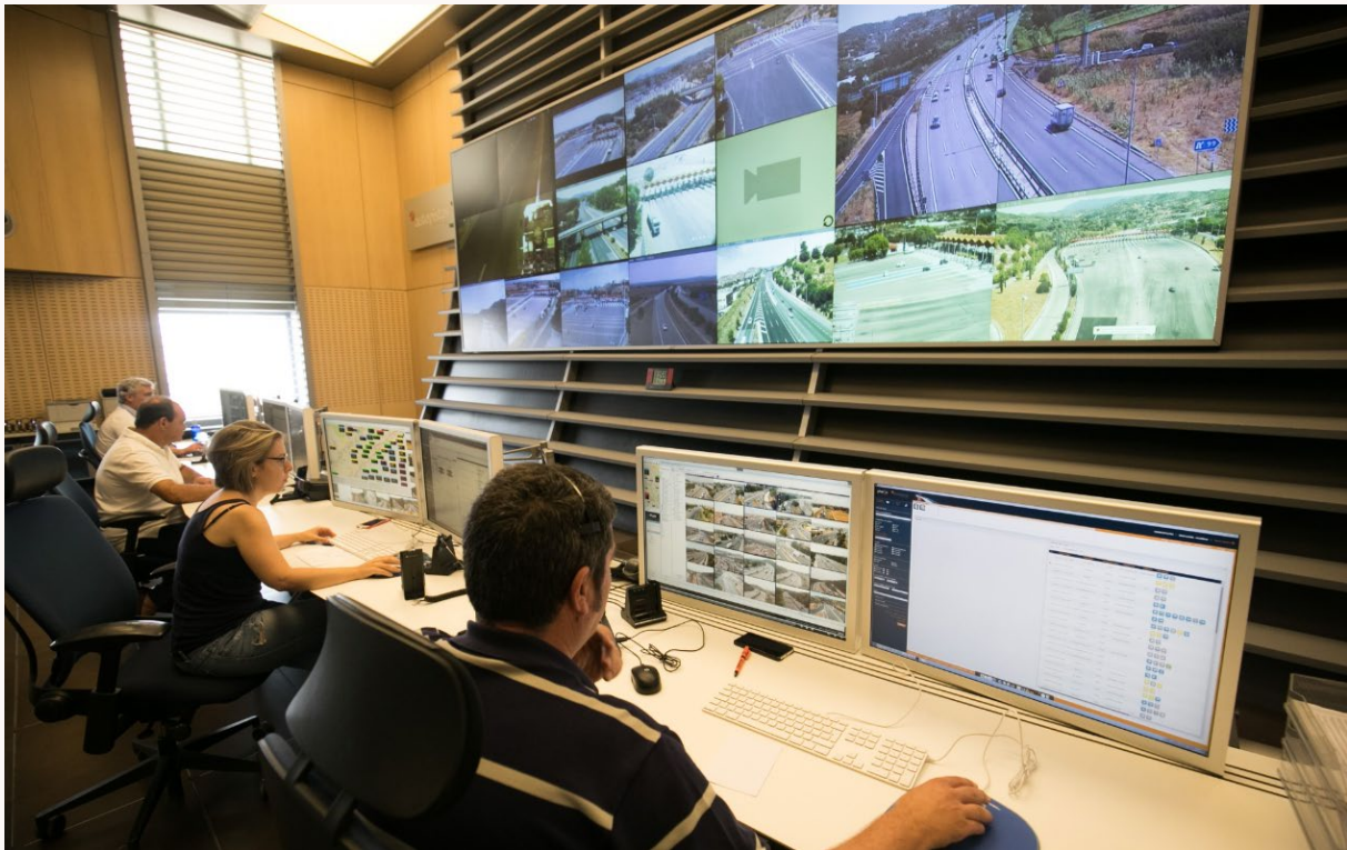
Illustration 62: Highway Operations and Road Safety Center. Source: Autopistas
