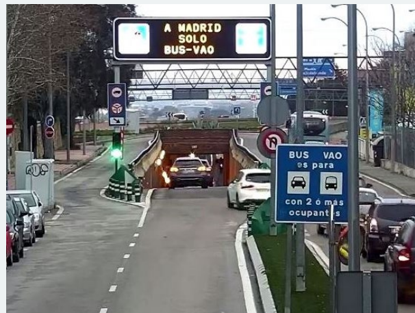
Illustration 26: HOV-Bus lane in A-6 access. Source: DGT
