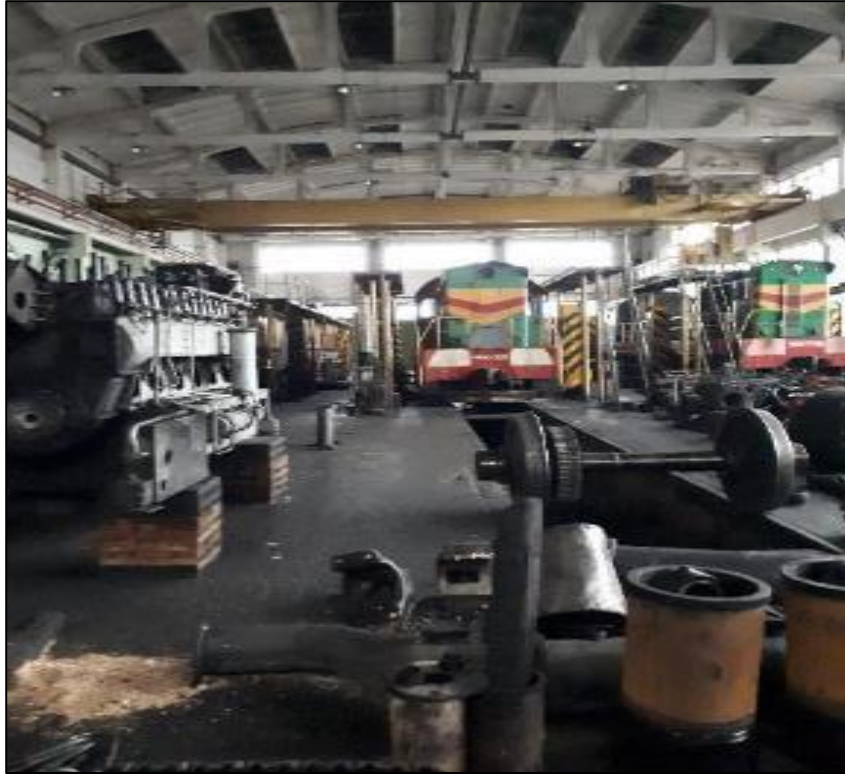
Figure 4.6: Old maintenance locomotive depot in Chisinau. Source: prepared for JASPERS by Egis
