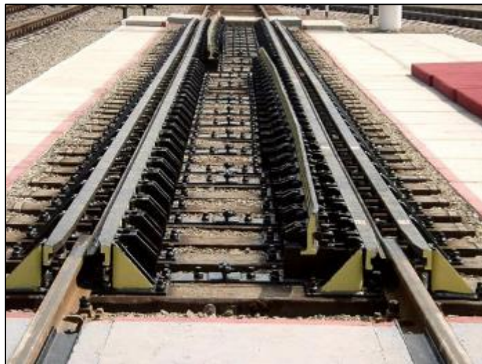
Figure 6.1: Gauge-changing facility. Source: prepared by Egis for JASPERS
